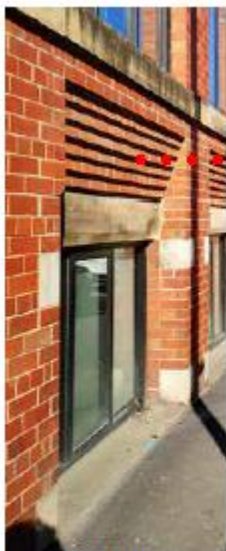
Brick detailing to openings - Britannia Mill
